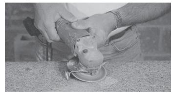
3.2 Clean and grind back of stone at areas to receive LATAPOXY 310 Stone Adhesive using a mechanical wheel grinder with a diamond wheel/blade. Remove dust with a stiff brush, wipe entire surface. Using a damp sponge (not wet), wipe the tile or stone to remove any particles or remaining dust to ensure a clean direct bond and that all ground material is removed. Wipe dry with a clean cloth, then apply LATAPOXY 310 Stone Adhesive.
